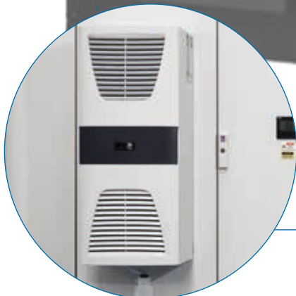
*COOLING UNIT AC TO COOL THE ELECTRICAL CABINET
